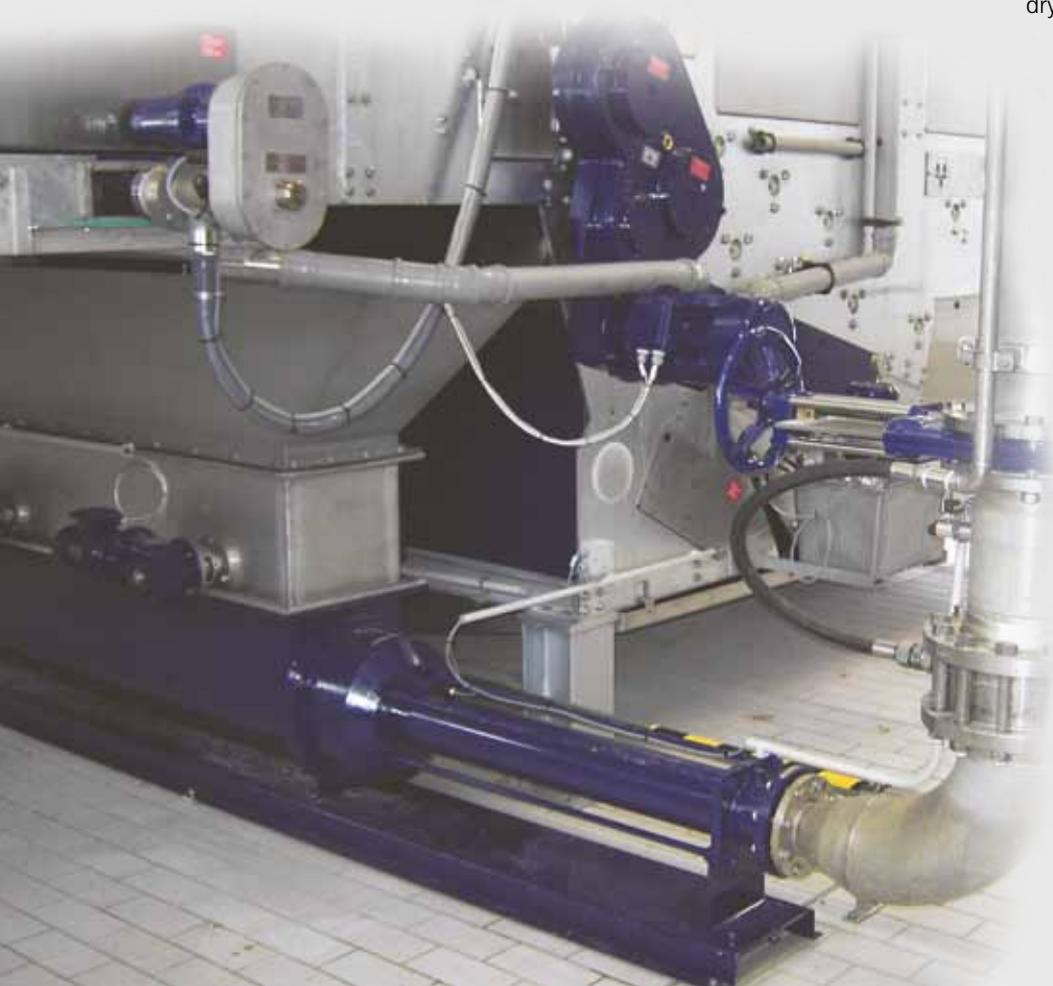
*NEMO® Sludge Cake Pump with customized 1.5 meter hopper pumping 20 - 22% dewatered sludge from a belt filter press to a drying plant 110 ft. (34 m) away. Pump employs dual aBP-Module (Asynchronous Bridge Preventing Module) and STP stator run dry protection system.*
