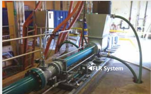
NEMO® Sludge cake pump with NETZSCH FLR System injecting 0.5 gpm (.11 m<sup>3</sup>/hr) of water into the pipeline to reduce pressures by about 50%. Dewatered sludge is conveyed over 75 ft (23 m) at 15–20 gpm (3.5–4.5 m<sup>3</sup>/hr). Additional flanges added to the hopper for cleaning of the pipeline and pump.
