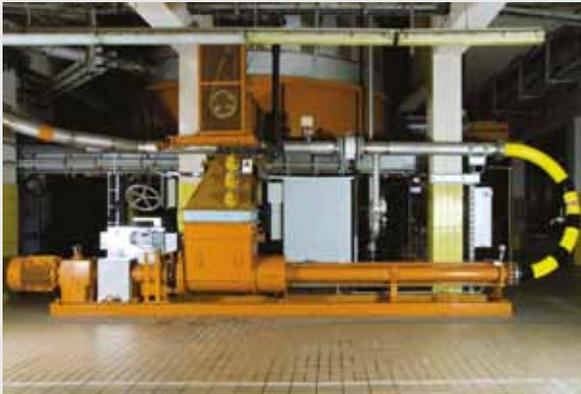
NEMO® Sludge Cake pump with bridge breaker conveying dewatered sludge immediately overhead via a long radius elbow 270 ft. (80 m) to incinerator. Solids content approximately 25%–32%, flow-rate of 8–60 gpm (2–14 m<sup>3</sup>/hr) at 360 psi (25 bar) discharge pressure.
