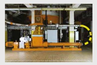
NEMO<sup>®</sup> Sludge Cake pump with bridge breaker conveying dewatered sludge immediately overhead via a long radius elbow 270 ft. (80 m) to incinerator. Solids content approximately 25%–32%, flow-rate of 8–60 gpm (2–14 m<sup>3</sup>/hr) at 360 psi (25 bar) discharge pressure.
