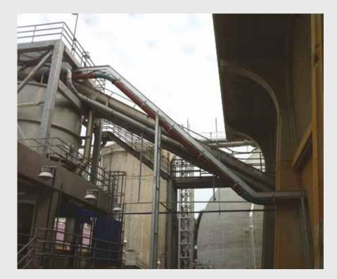
In the foreground is the new closed conveying system with vertical piping discharging into a storage tank. Immediately behind it is the open auger system that has been discontinued.
